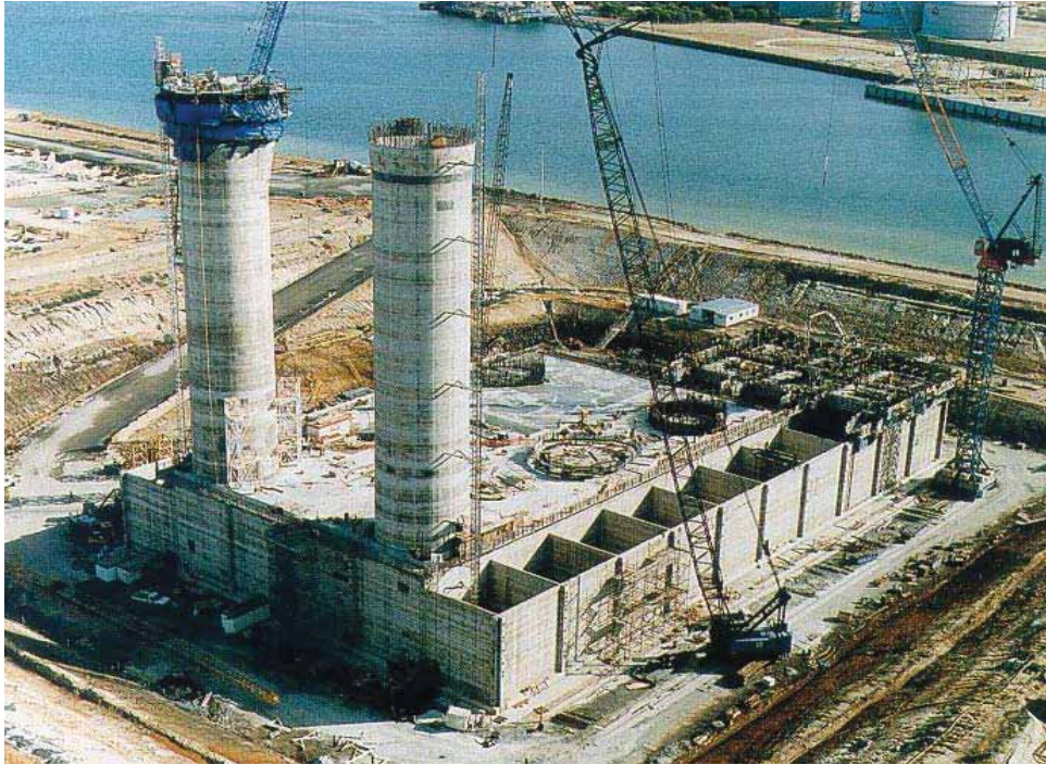
Figure 6. Concrete caisson for the Wandoo offshore oil field, Australia
