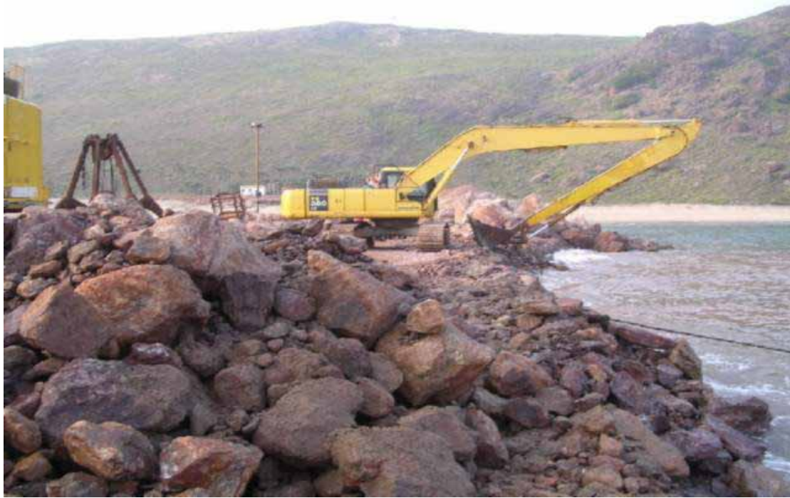
Example of a rock embankment under construction
